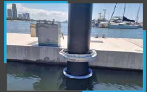
PILE RING IN ACTION
